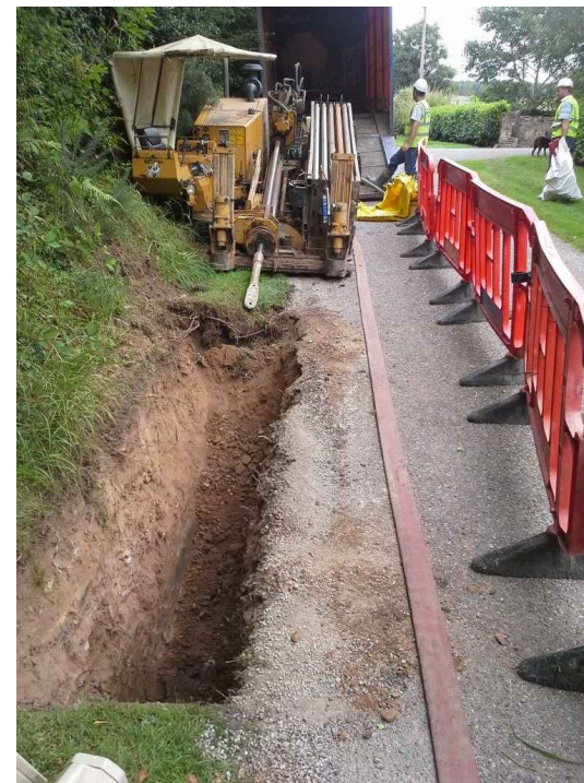
Typical Drilling Rig & Launch Pit
